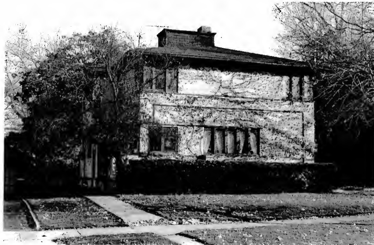
The arrangement of window openings and wood trim on the H. Howard Hyde House betrays the block-like form of its massing and plan.
